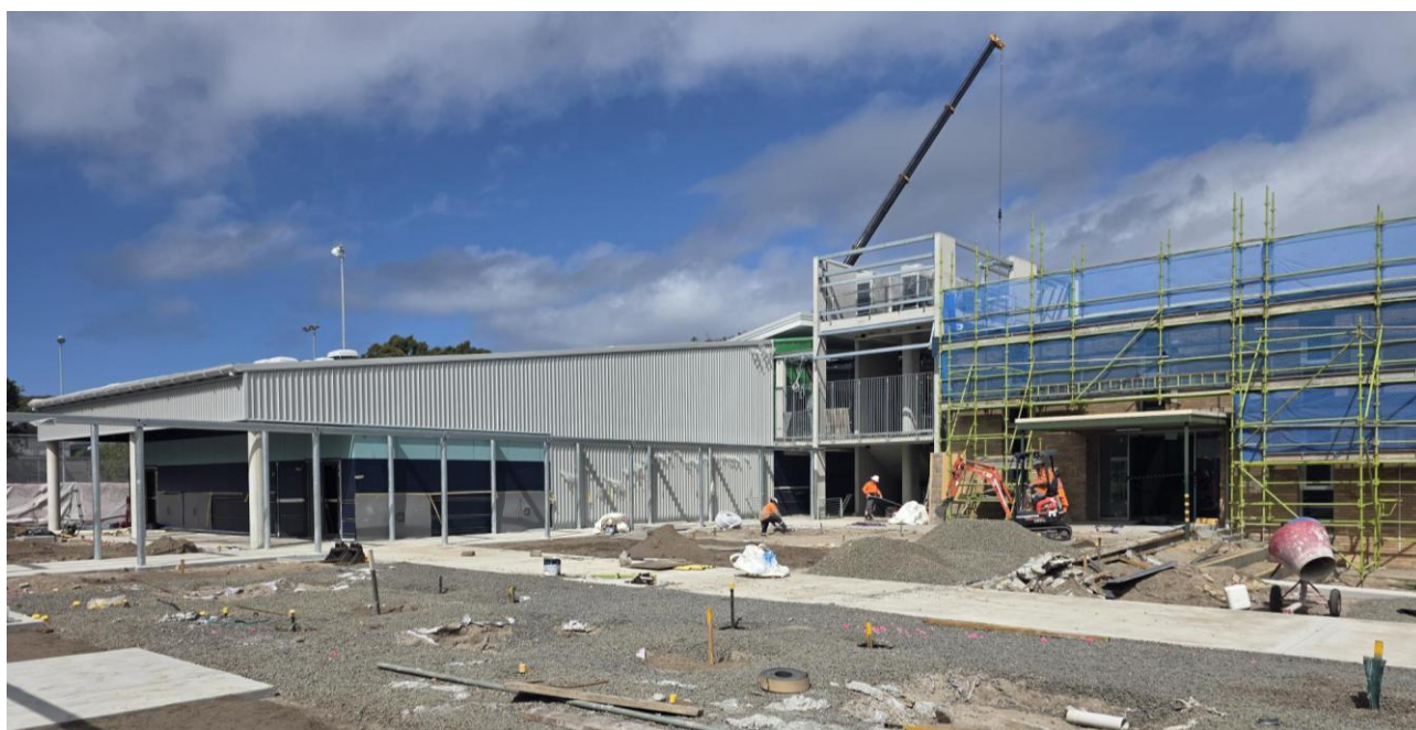
Progress photo of new lecture theatre (left) and performance hub (right)
